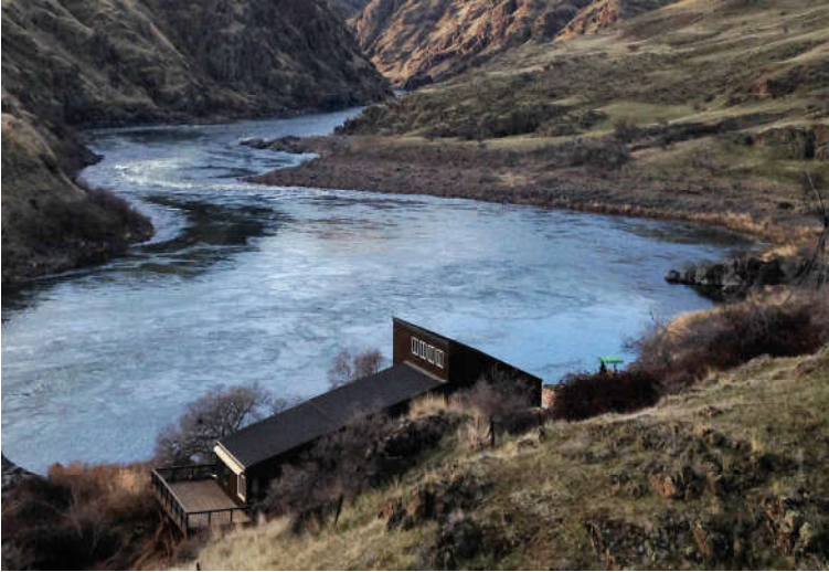
*Picture is before solar array addition
