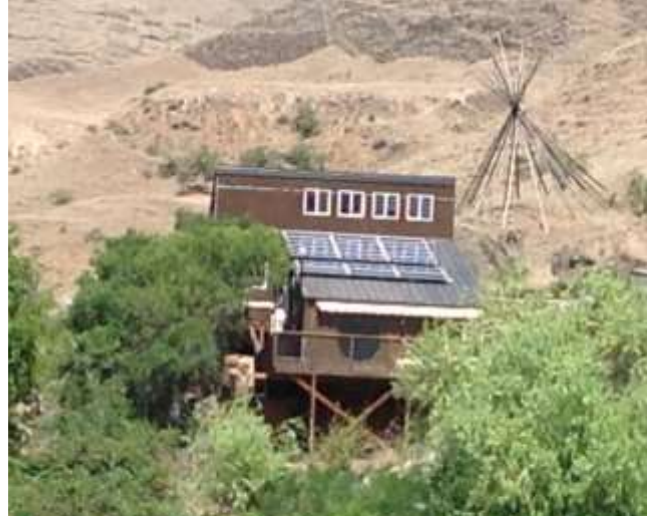
*Picture including Solar Panel Addition
